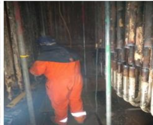
Inside the Boiler removing and fitting 2.25% Chrome boiler Tubes
