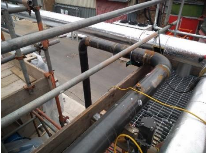
2.25% Chrome Boiler Pipework
