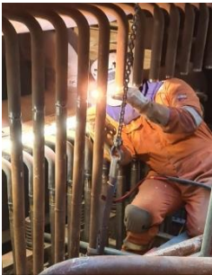
Welding Superheater Tubes
