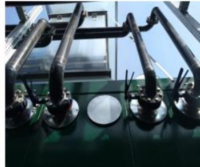
High Pressure Pipework from the Boiler
