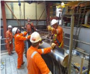
Boiler Headers and Superheater panel being lowered into place
