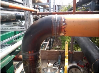
2.25% Chrome Boiler Pipework
