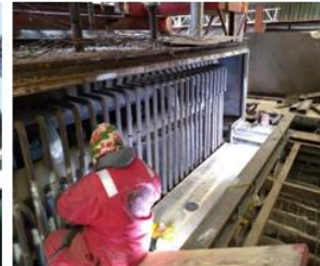
Preparation of Superheater Tubes
